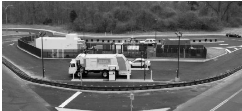
Figure 26. Hauppauge fast-fill compressed natural gas station
